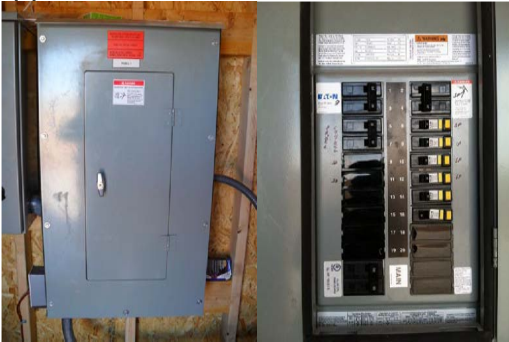
Figure 15 - Master power controls
