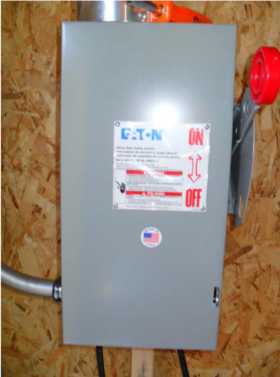
Figure 22 - Battery shut-off
