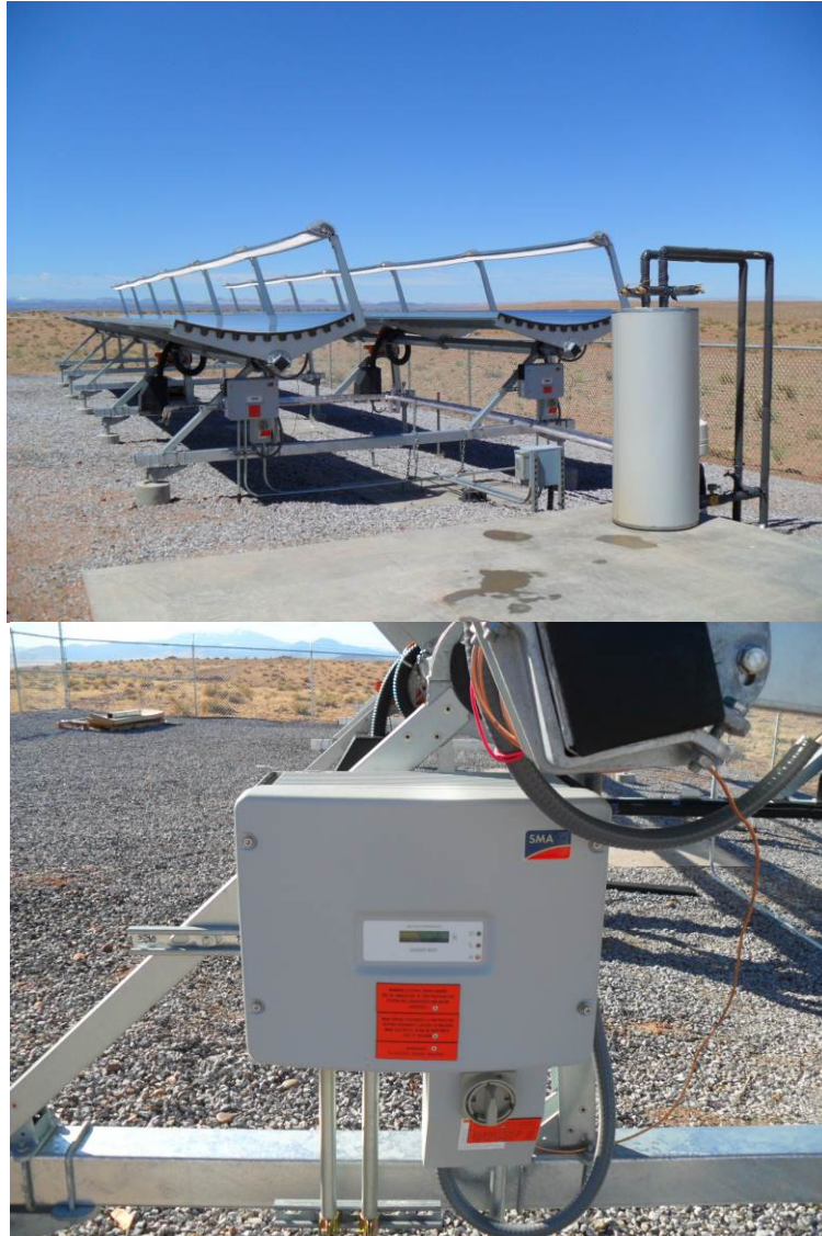
Figure 18 - Sunny Boy inverters
