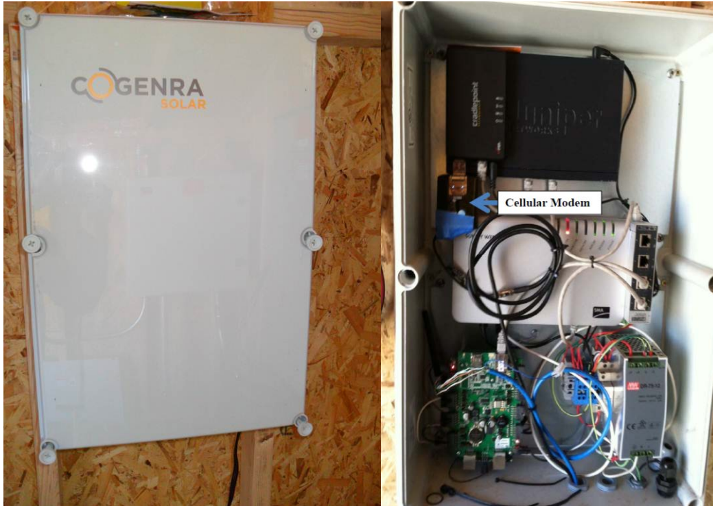
Figure 19 - Communication cabinet
