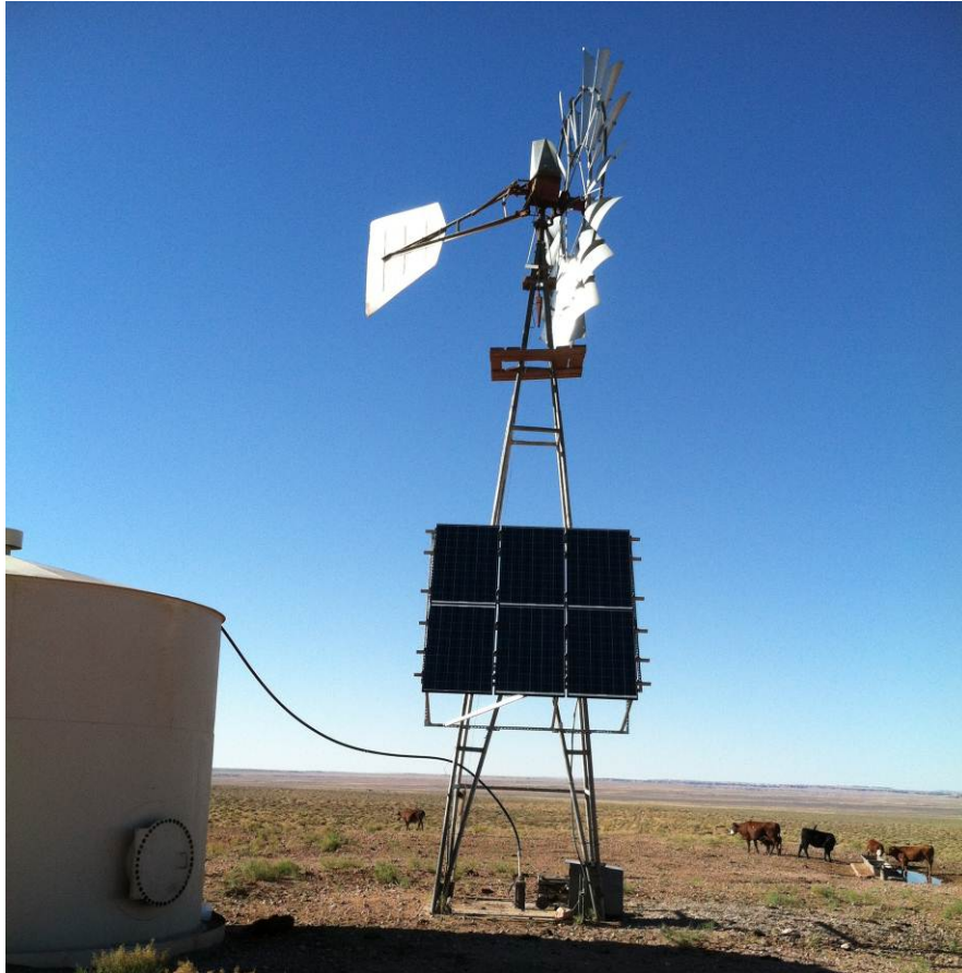
Figure 10 - Dedicated solar panels for pumping
