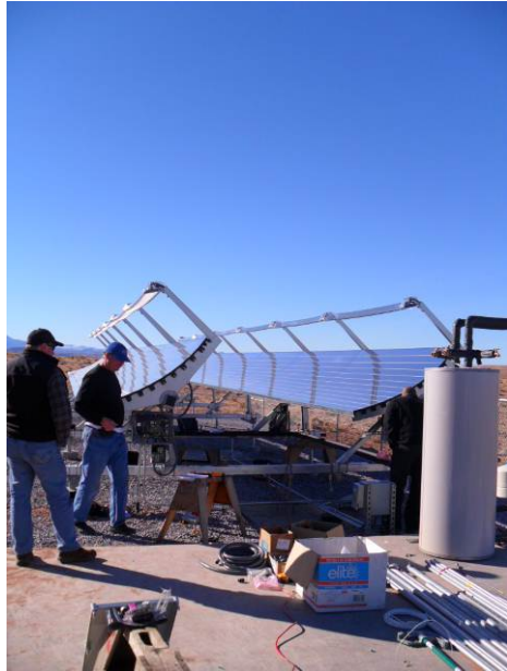
Figure 13 - Constructing the CPVTHS
