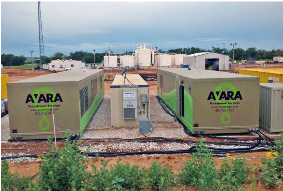
Purestream Services commercial operations deployment March 2014 to treat Eagle Ford Shale produced and flow-back water In Gonzalez County, Texas (Avara, used by permission).
