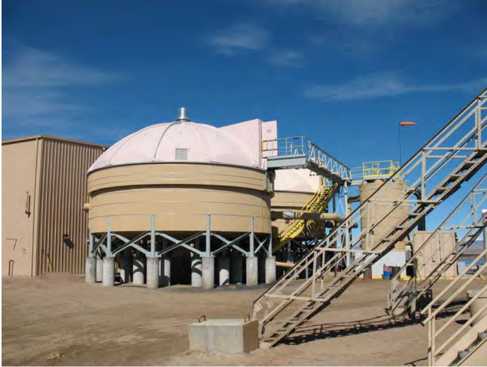
Exterior facility shot focusing on one of the two large dissolved air flotation units (NGL Water Solutions, used by permission).
