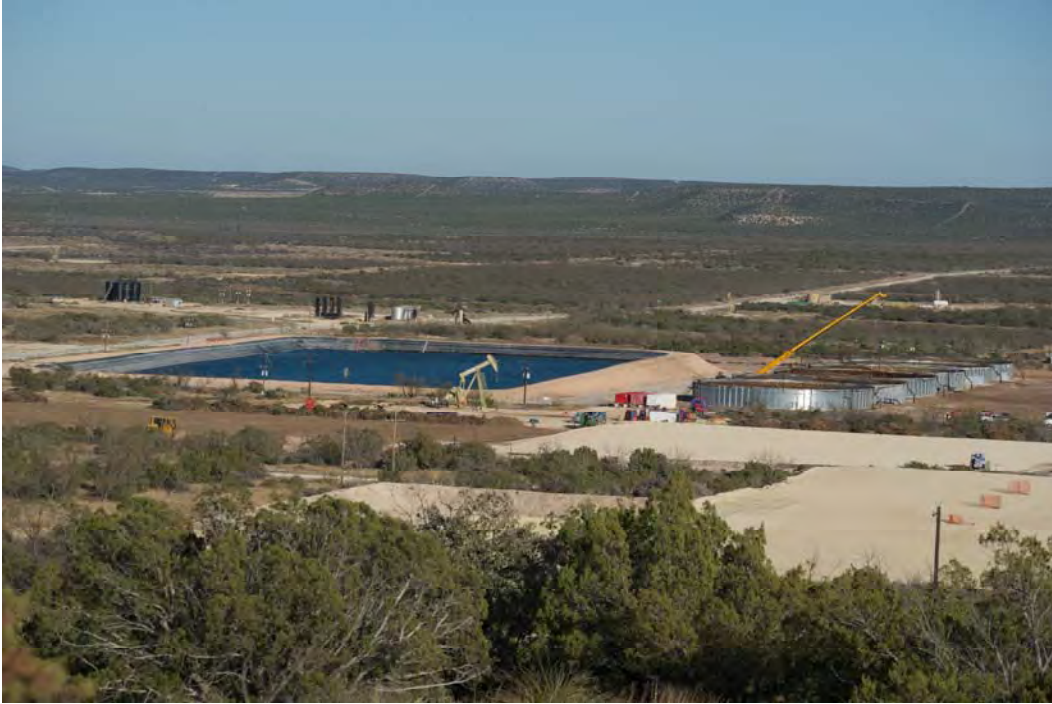
Apache Corporation uses non-potable brackish water from the Santa Rosa aquifer and recycles produced water to supply all of the water needed for well completions in the Barnhart area. The re-engineered grain bins are used to treat produced water before it is reused (Apache Corp., used by permission).
