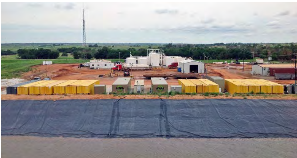
Purestream deploys AVARA vapor recompression systems to Eagle Ford to treat 2,500 barrels per day for reuse (Avara, used by permission).
