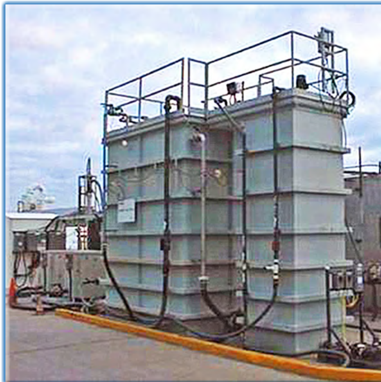
Kruger Neosep membrane bioreactor system at San Diego Pt. Loma WWTTP (Reclamation photograph).
