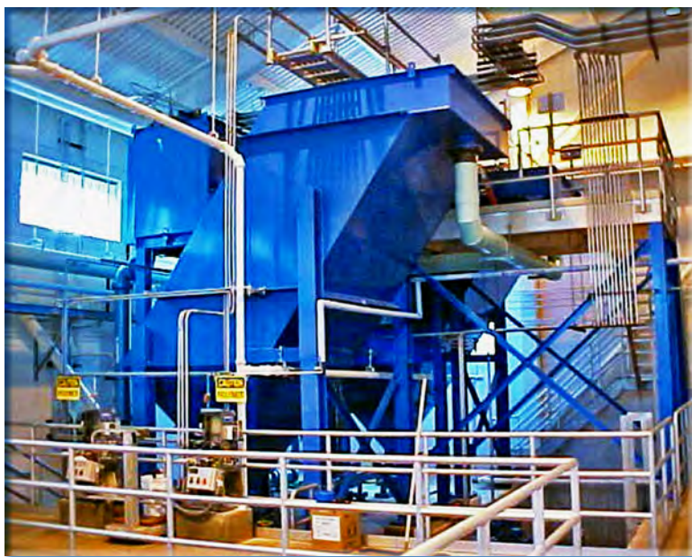
Inclined plate settler (Parkson Corp., used by permission).
