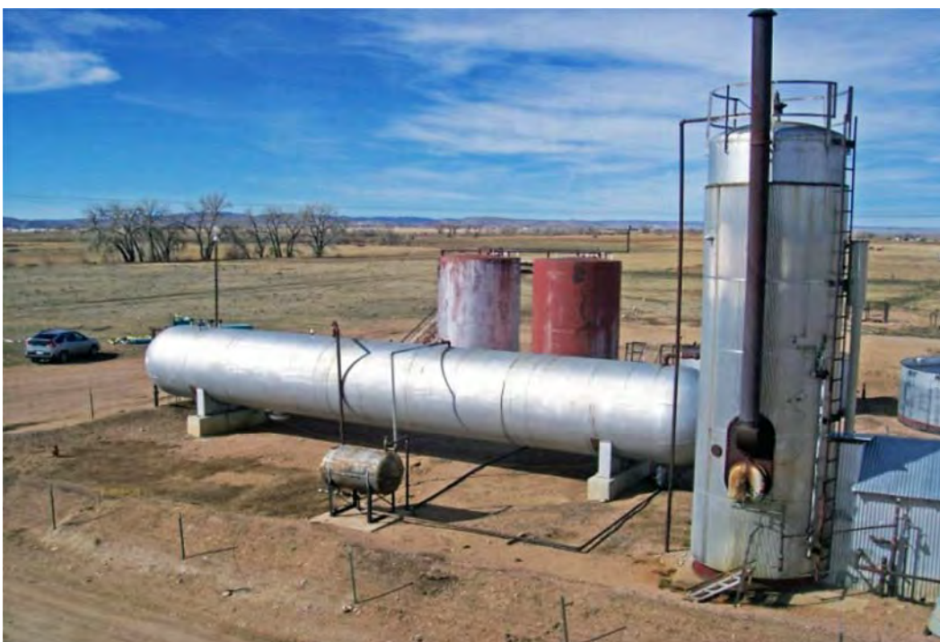
Oil/water separator at the Wellington Operating Site. (Stewart Environmental Consultants, Inc., used by permission).
