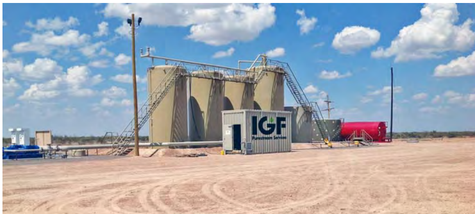
IGF Plus technology can treat anywhere from 2,500 to 80,000 barrels per day. It is commonly used in offshore platforms and removes suspended solids and oil and grease to 1 micron, but does not remove chlorides. Producers are able to re-use the treated water to frack with; typically it can treat water for under $.75 per barrel (Purestream, Inc., used by permission).
