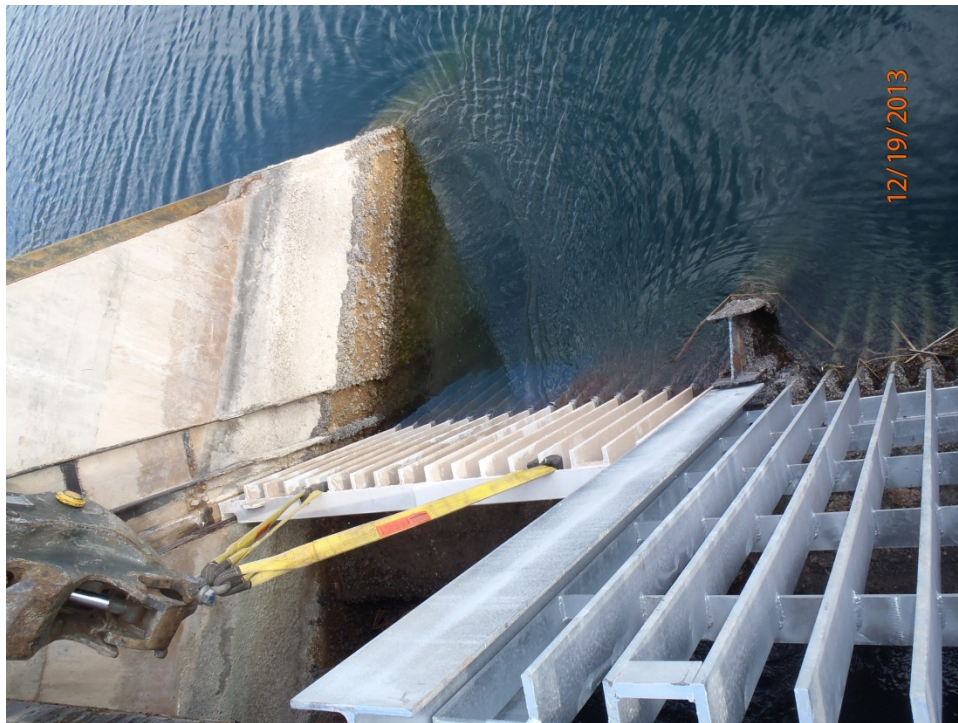
Figure 6.—Installation of the new trashrack panel.
