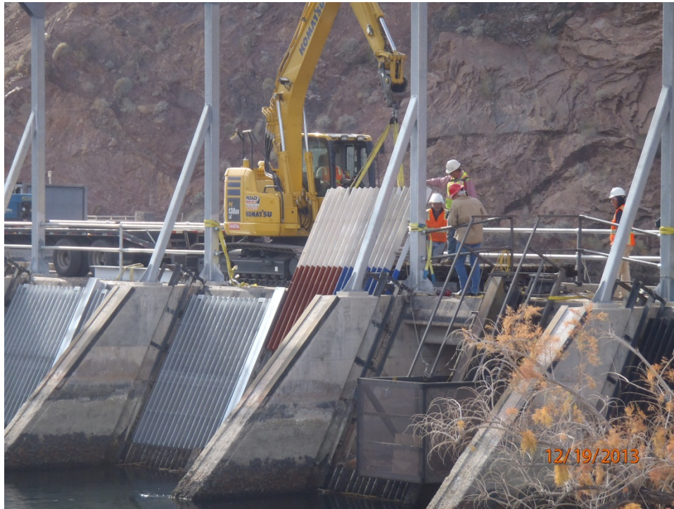
Figure 5.—Installation of the new foul release coated panel.
