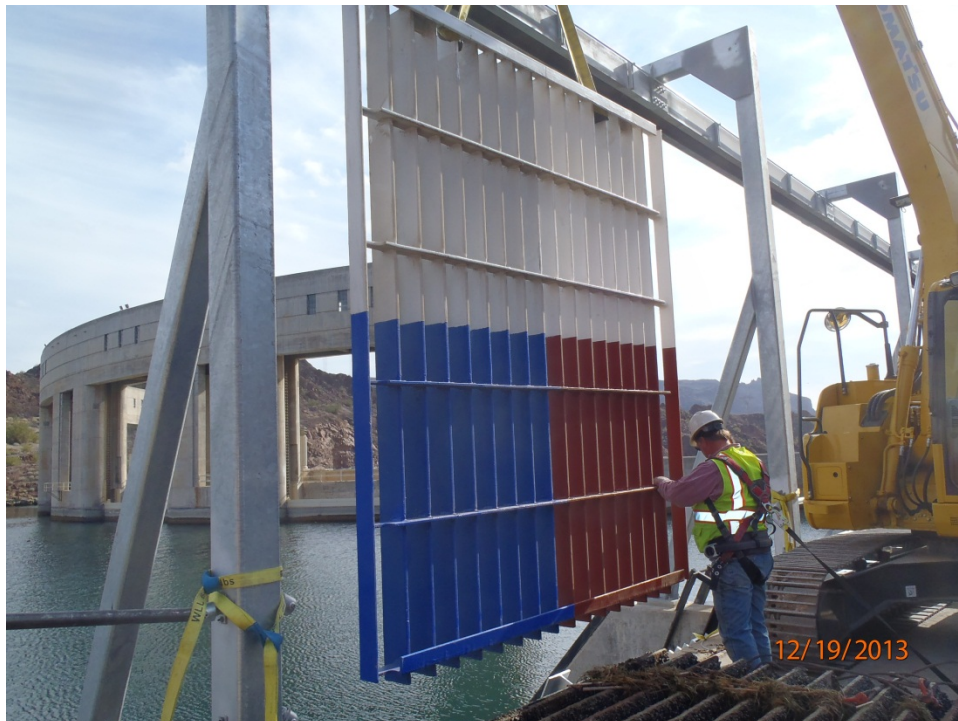
Figure 4.—Installation of the new trashrack panel.
