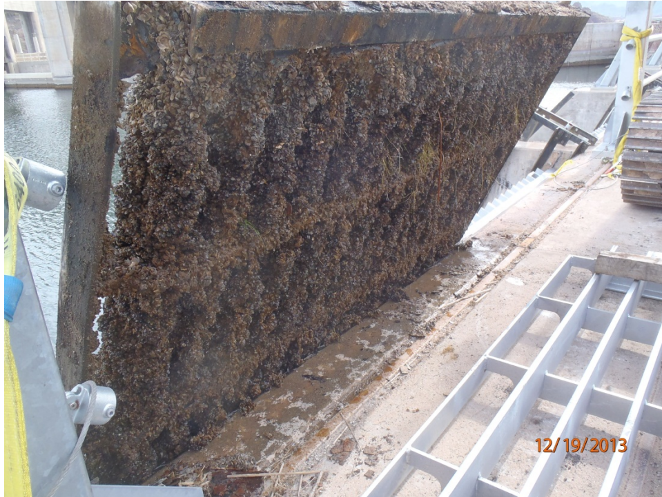
Figure 1.—Existing trashrack heavily fouled with quagga mussels.
