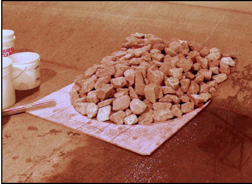
Figure 3.18: Plywood Shape Template for Weir Construction
