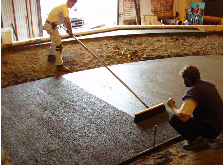
Figure 3.6: Installation of the concrete cap in the Middle Rio Grande model.
