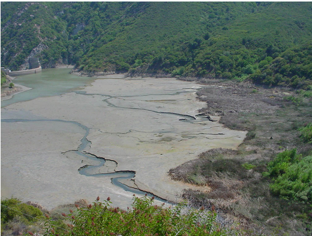
Figure 14. Picture of sediment trapped behind Matilija Dam while the reservoir was drawn down. Picture was taken in July 2003 by Paul Jenkin of the Surfrider Foundation.
