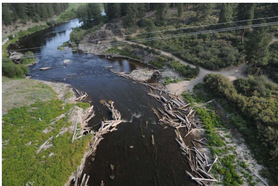
Figure 28. Looking at Chiloquin reservoir following removal showing the large number of logs that were uncovered.
