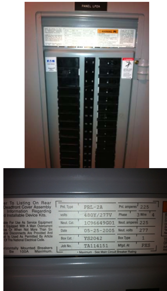
Figure 26 - Panel LP2A has many spaces where PV breakers could be installed (top); 225 A, 480 V Panel LP2A has adequate capacity for PV (bottom)
