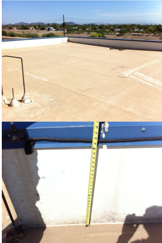
Figure 25 - East wing roof looking east (top) is also suitable for PV (750 ft 2 ); typical parapet is about 28-inches high (bottom)
