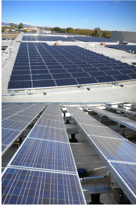
Figure 23 - Typical Ballasted PV System at GSA Denver Federal Center
