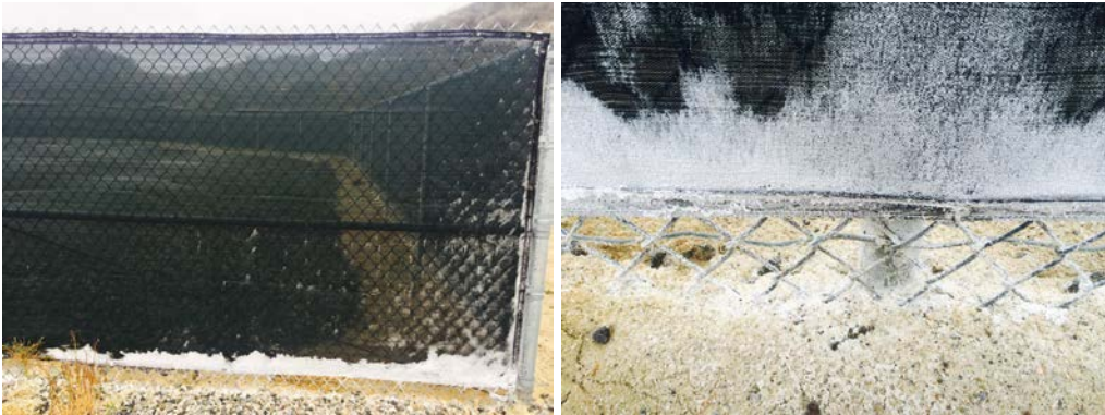
Figure 16.—Accumulation of solids along fence line.
