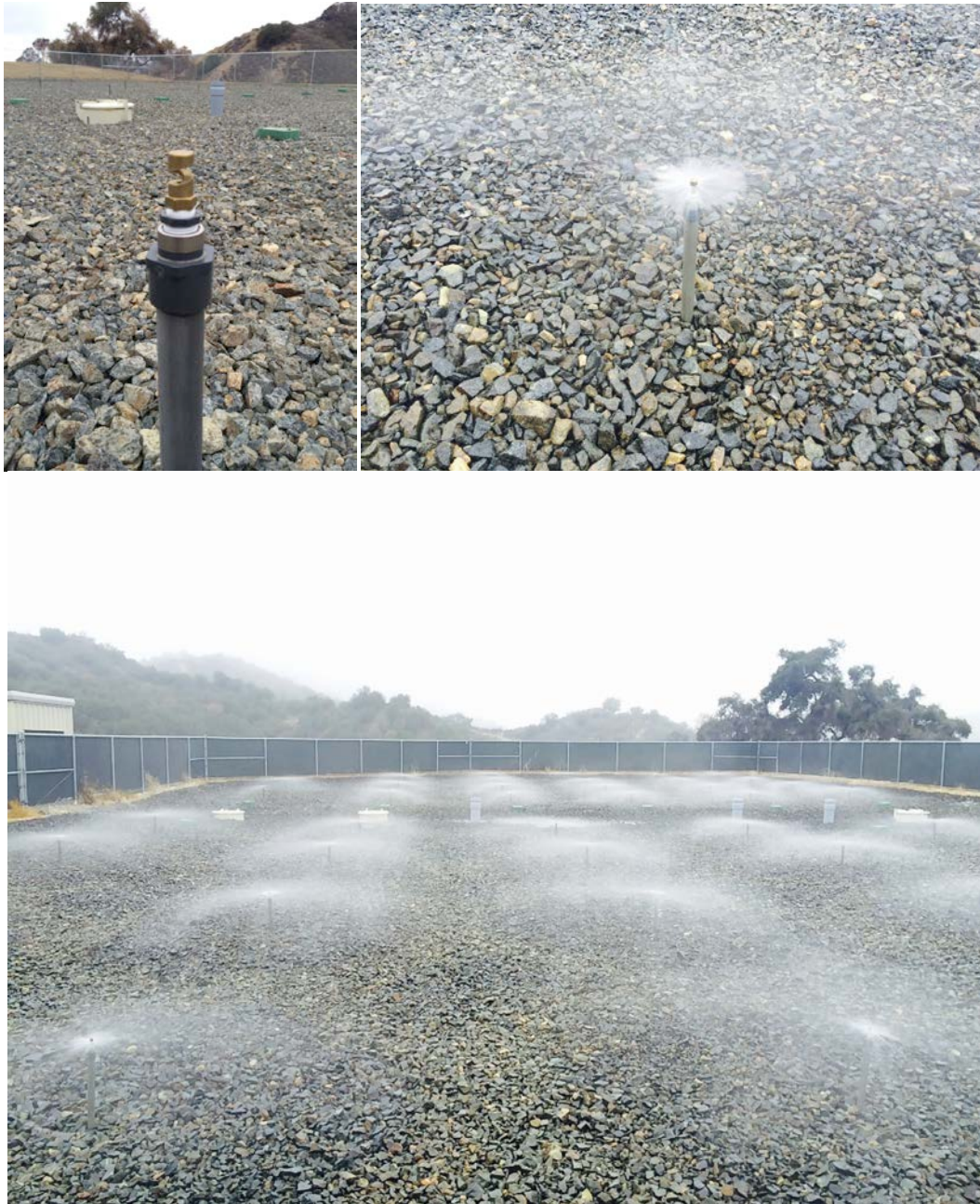
Figure 9.—High rate solar evaporator bed and nozzle
