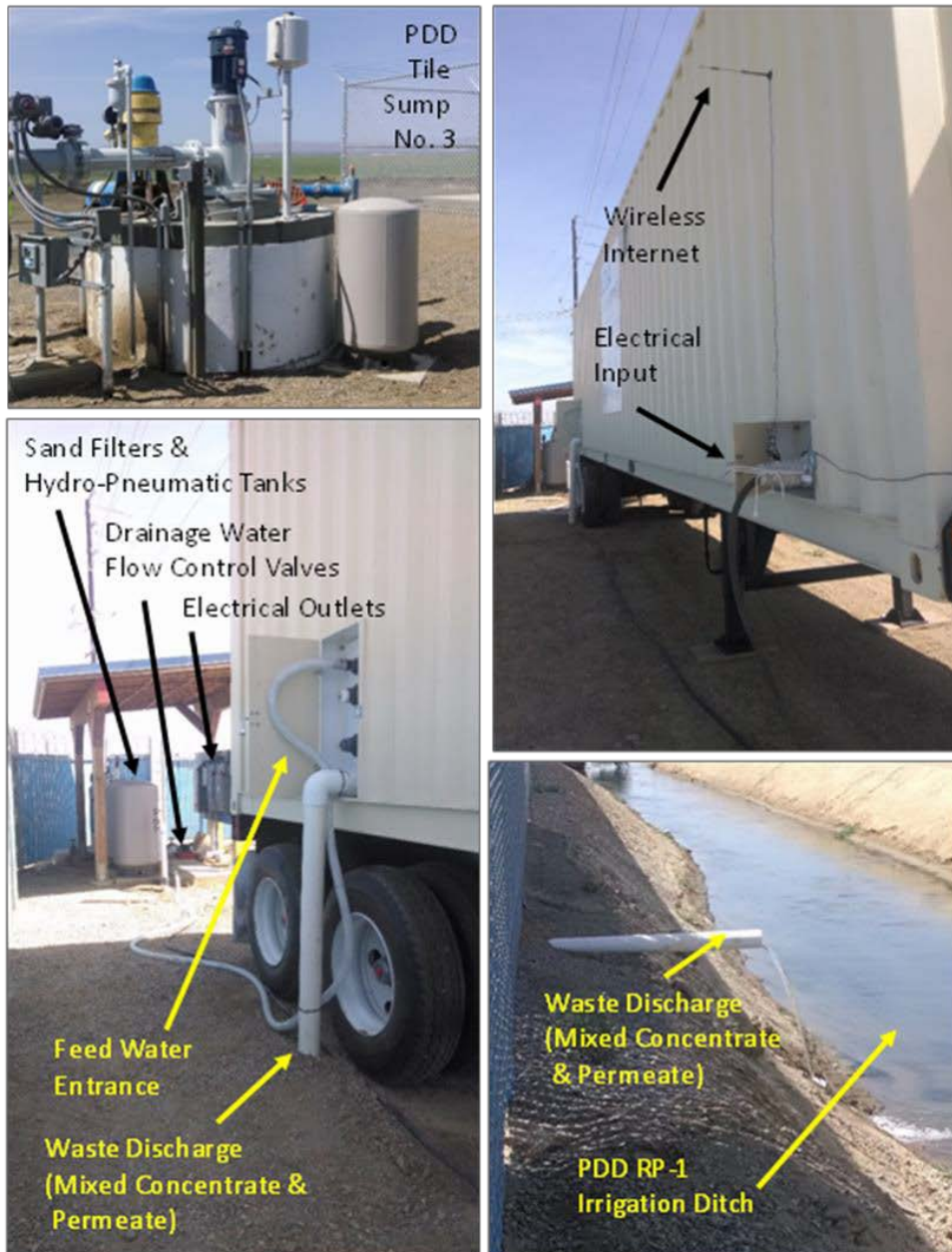
Figure 14. Field infrastructure at Panoche Drainage District treatment site, supporting operation of the UCLA desalination mobile unit.
