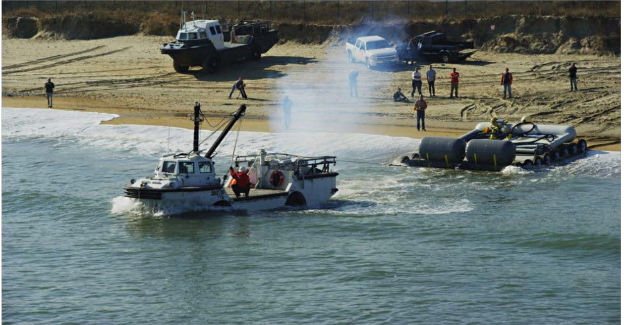
Figure 30. Beach Launch and Deployment of SurgeWEC.
