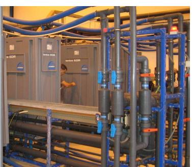
Figure 2-3 Electrodialysis Reversal Desalination Equipment in Gran Canaria, Spain
