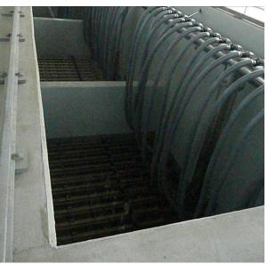
Figure 2-11 Submerged configuration membrane filtration (Siemens Water Technologies)
