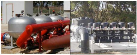
Figure 2-15 Spin Klin modularity allows for a wide range of system layouts
