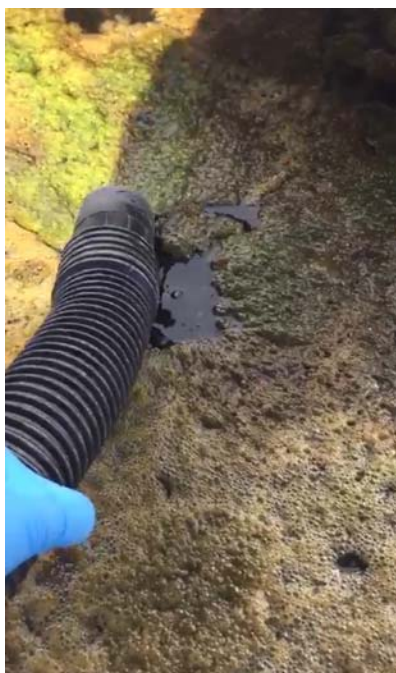
The green floating biomass from Channels 3 – 9 was removed using a vacuum cleaner.
