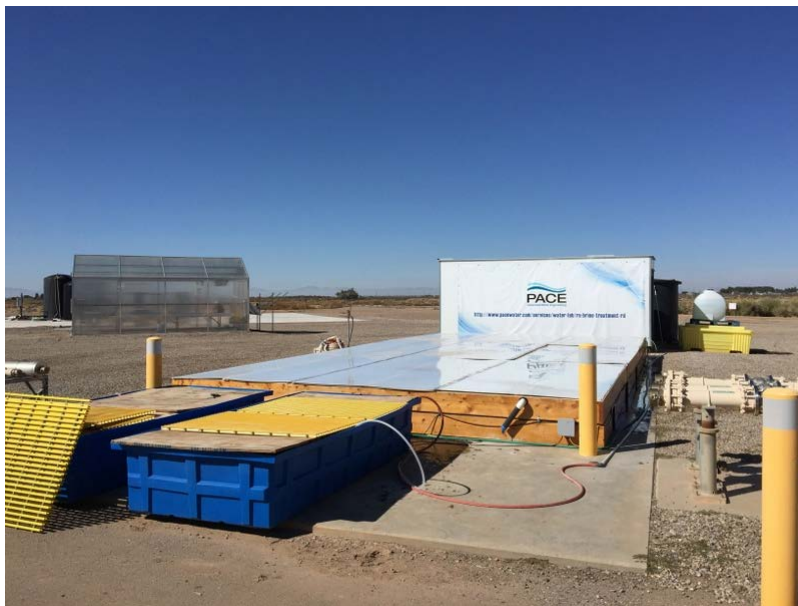
Figure ES-1.—1,500-Gallon (5,700-L) Pilot-scale Photobioreactor at the BGNDRF.
