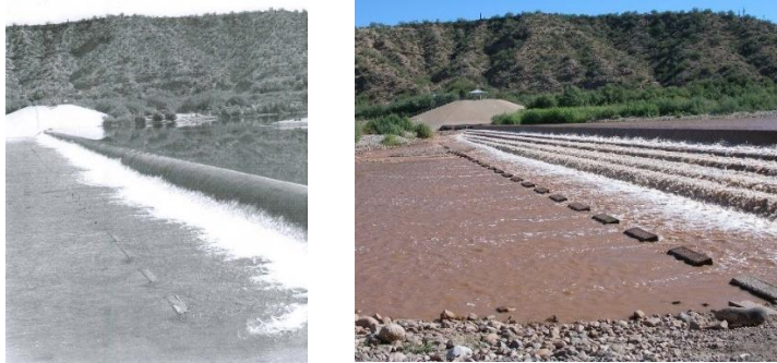
Left: Original ogee-shaped weir design of Reclamation's Power Canal Diversion Dam upstream of Roosevelt Dam.
