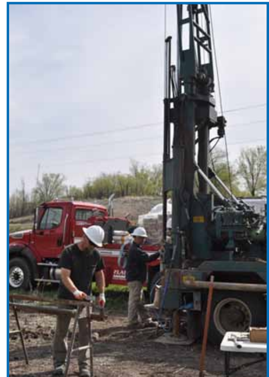
Drillers and the rig obtaining core samples.
