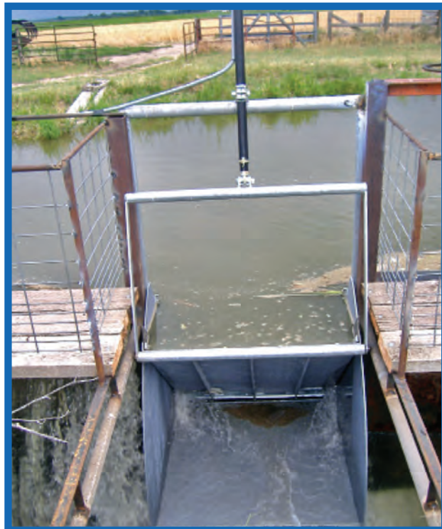
Overshot gate at South Platte Ditch Company, Colorado.
