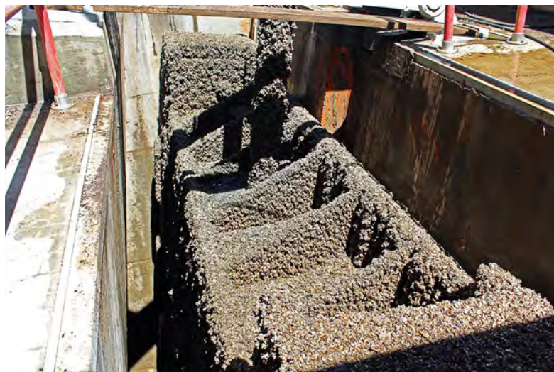
Quagga mussel fouling on a fixed wheel gate at Glen Canyon Dam.
