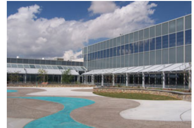
El Paso Desalination Plant Research Bay
