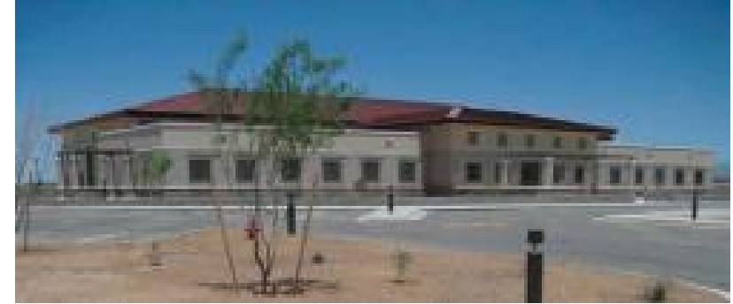
Brackish Groundwater National Desalination Research Facility Alamogordo, New Mexico
