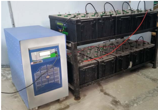
Batteries and inverter
