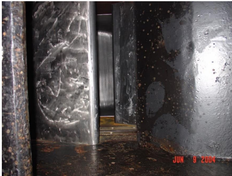
Photo 5.—Wicket gates and stay vanes.
