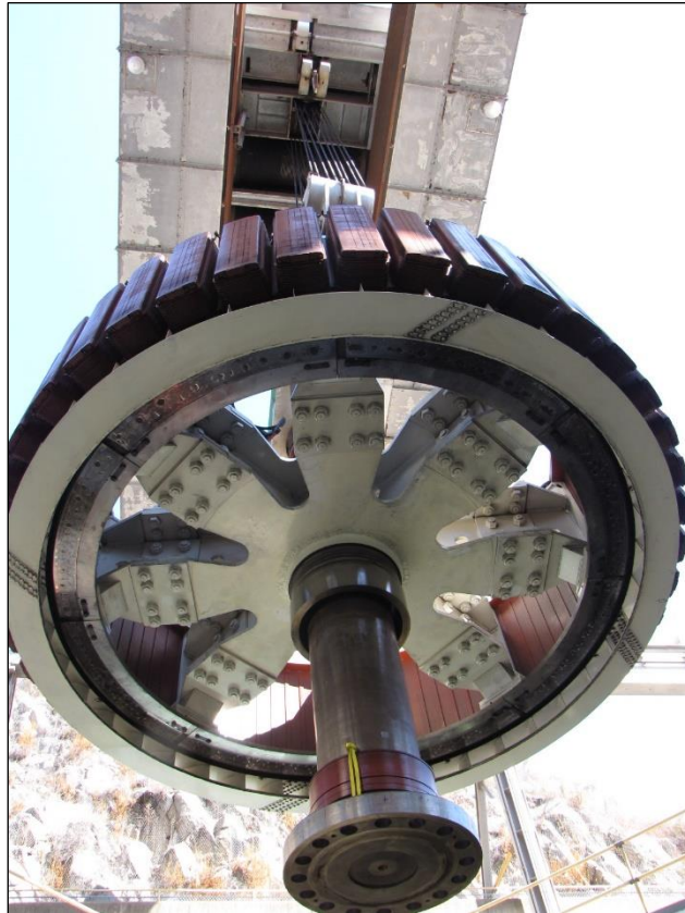
Photo 18.—Rotor assembly.
