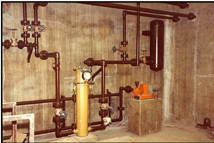
Photograph 11. Construction of the oil transfer system piping assembly.
