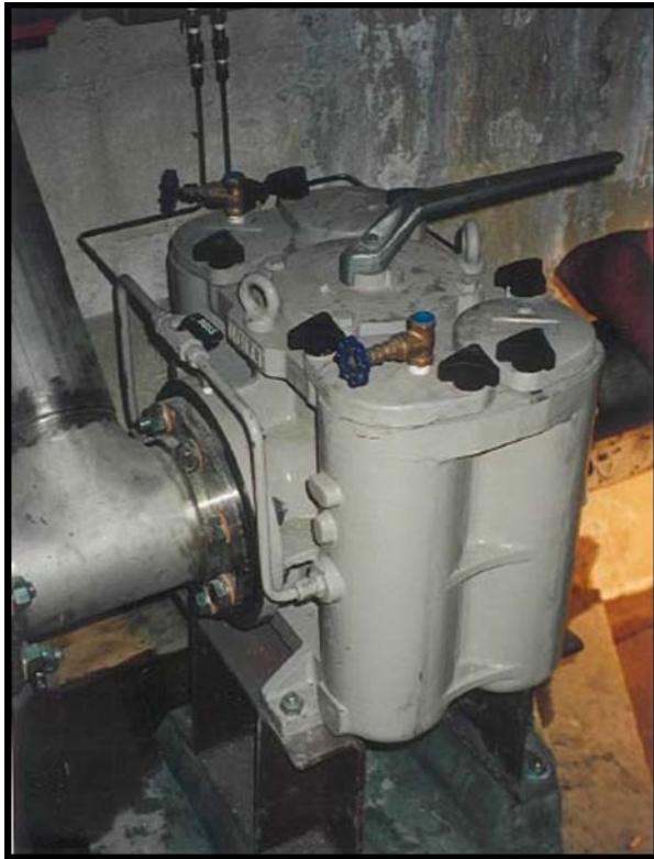
Photograph 6. Manual basket duplex strainer.
