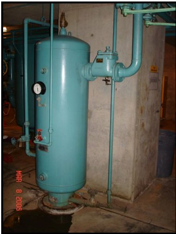
Photograph 12. Brake air receiver tank.
