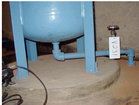
Pressure Vessel Mounting Supports
