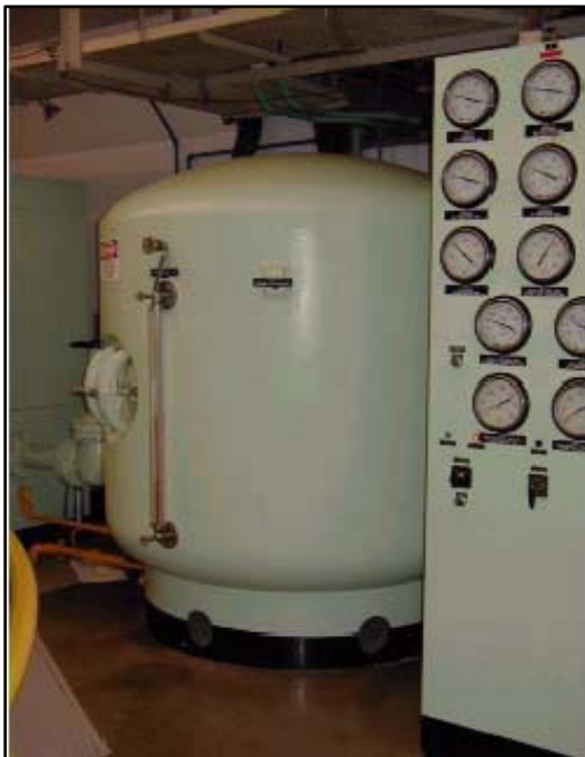
Photograph 1. Governor Oil Tank
