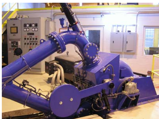
500 kW Canyon Pelton Turbine for Colorado Springs Utility
