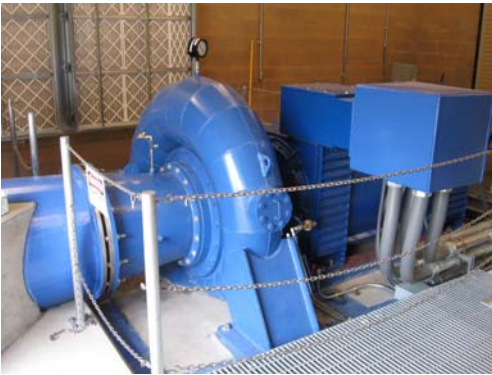
720 kW Canyon Francis for Swalley Irrigation District, Ponderosa Hydro
