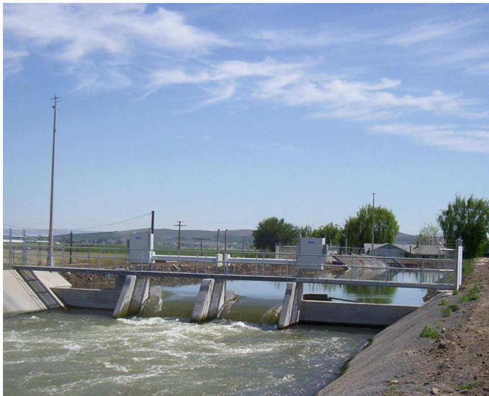
Figure 3. Langemann Gate – source Aqua Systems 2000 web page - Langemann® Gate | Aqua Systems 2000 Inc.
