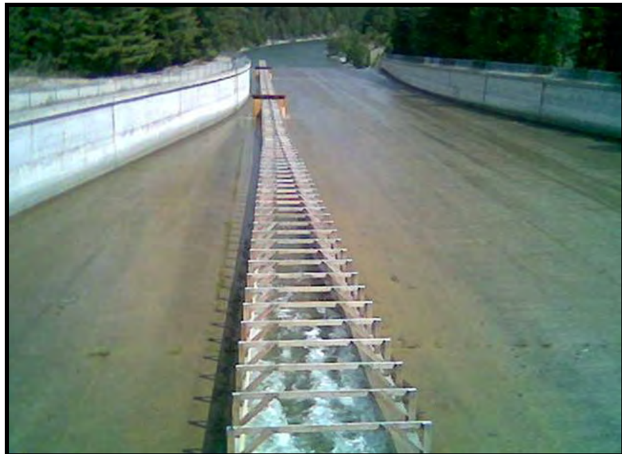
Photo 4. Fish passage flume and PIT tag antennas
