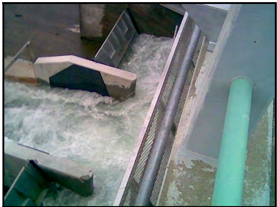
Photo 2. Plunge pool and entrance to flume
