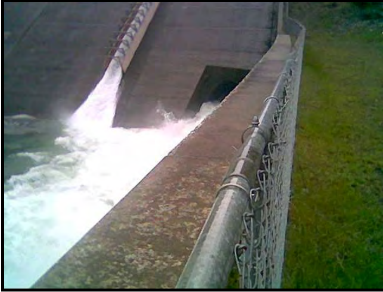
Photo 7. Fish passage flows and outlet works releases looking upstream
