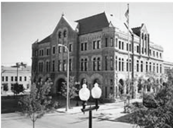
US District Courthouse, Sioux Falls, SD
