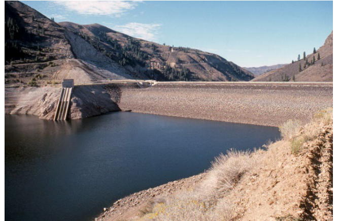
Anderson Ranch Dam and Reservoir
