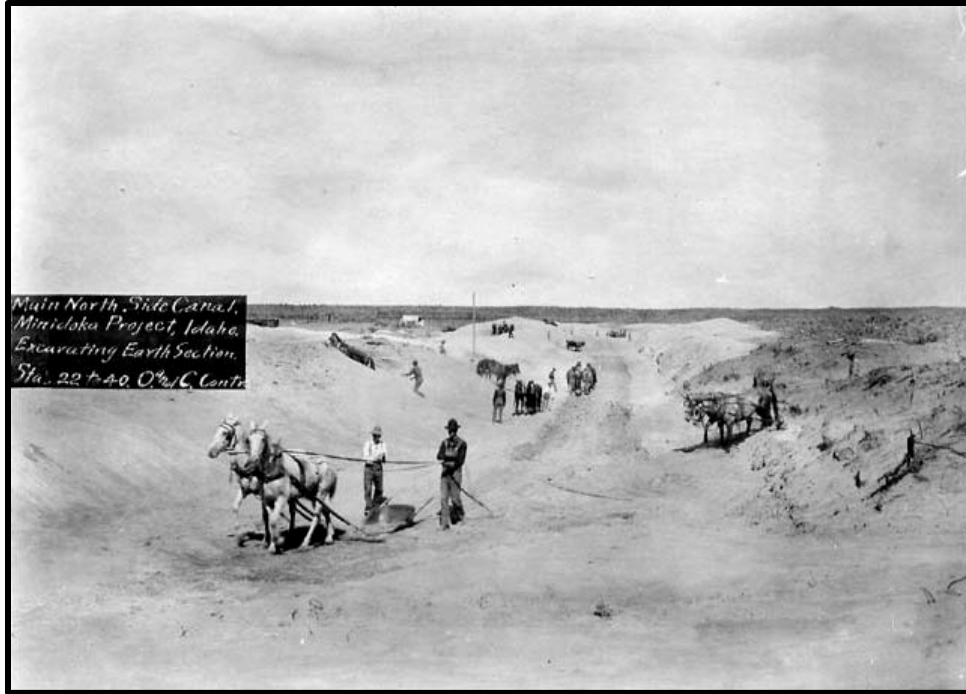
Figure 3. Main North Side Canal, Excavating Earth Section, c.1905. Minidoka Project, Idaho. Reclamation Photo No. P17-100-4018.
