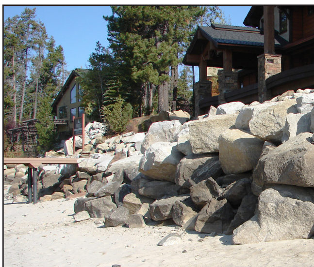
Example of stone rip-rap revetment.
