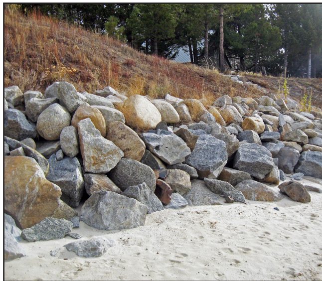
Retaining wall using large boulders and vegetation.
