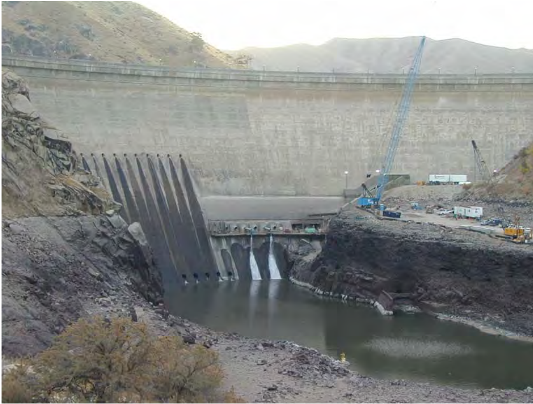
Figure 14. Middle and lower ensign valves at Arrowrock dam. Spillway is not shown and is located on the downstream right at the surface level of Arrowrock reservoir full pool.
