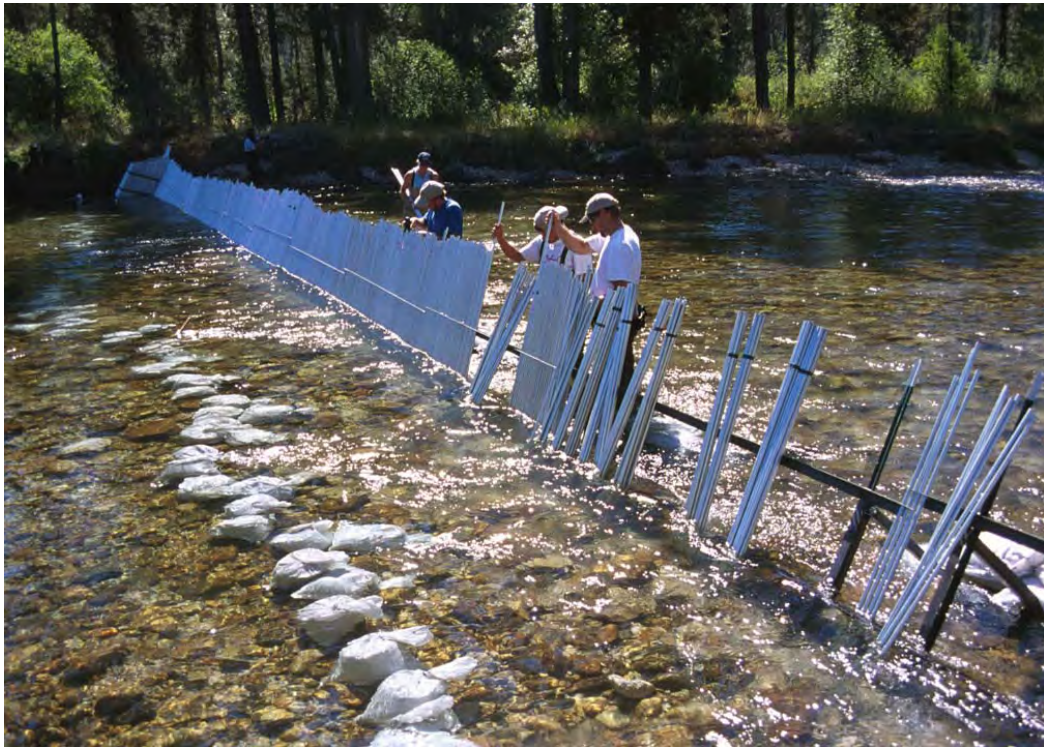
Figure 2. Installation of the North Fork weir trap. Steel frames, pickets, fence posts, and sand bags used for weights, to prevent channel undercutting, and escape by digging are shown.
