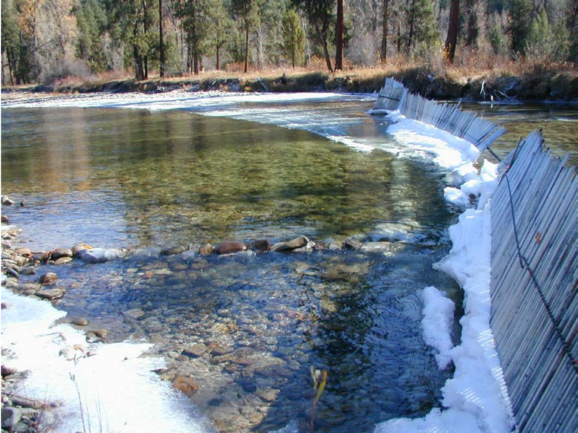
Figure 2. North Fork Boise River weir after snow and ice storm, 11/01/03
