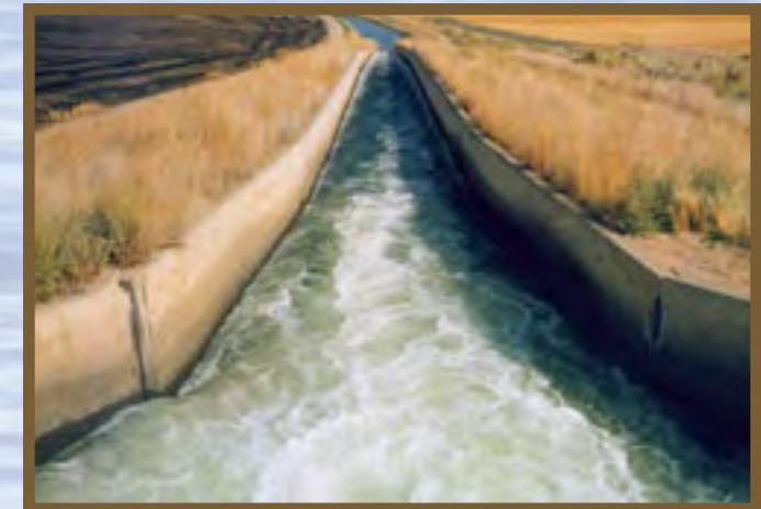
Water travels through both lined and unlined canals
