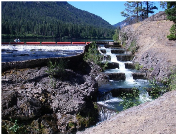
Pool-and-weir fish ladder in upper spillway channel
