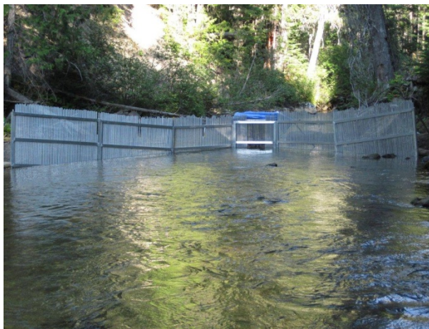
Completed picket-weir and box trap
