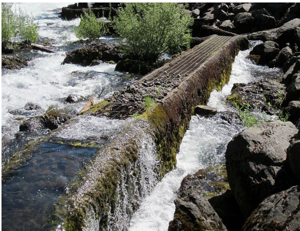
Upstream terminus of the Denil ladder completely clogged with cobble and gravel
