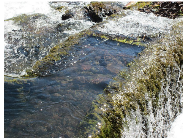
Upstream terminus of the Denil ladder completely clogged with cobble and gravel
