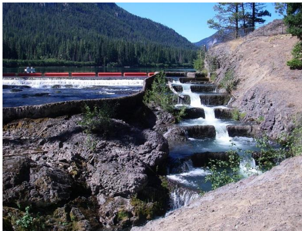
Pool-and-weir fish ladder in upper spillway channel
