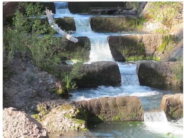
Pool-and-weir fish ladder in upper spillway channel
