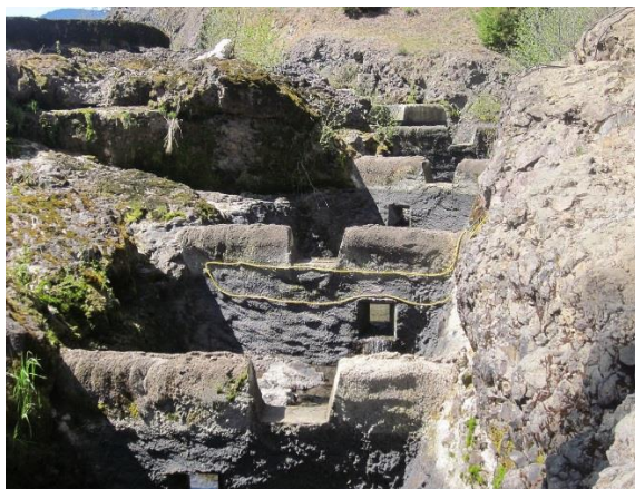
Lower ladder PIT tag detection antenna
