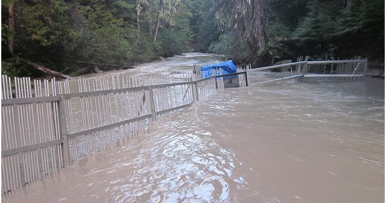
Figure 3. NF Tieton River fish trap after the high flow event on September 22, 2013. The photo was taken the next day after the river had receded.
