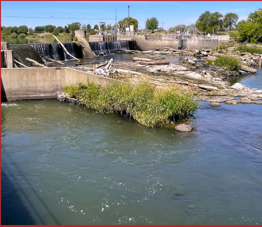
Prosser Dam at low flow. Picture taken from the right bank looking upstream at the dam. Fish Ladder entrance left of clump of grass.
