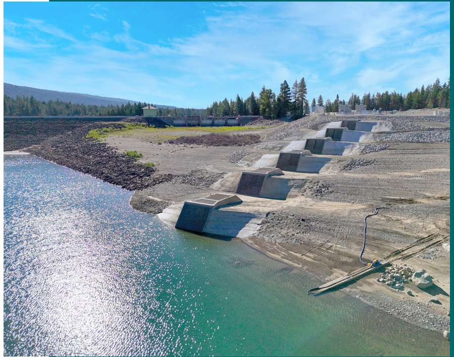
Intake gates at the Cle Elum Fish Passage Facility. These gates will help juvenile fish pass from the reservoir into the Cle Elum River.
