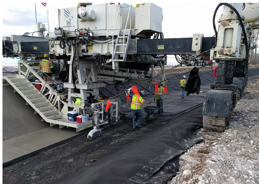
Construction workers lining KRD canals.
