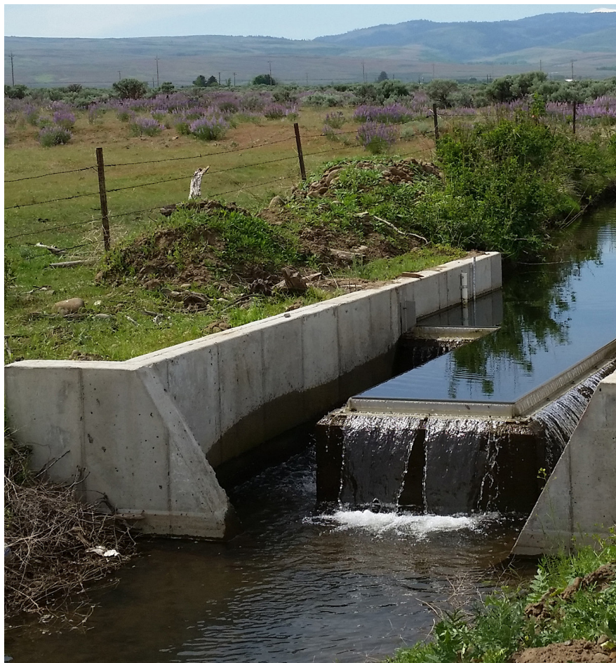
Mission Ditch is one of structures in a system of ditches and canals that reconnects channels to recharge groundwater in the Toppenish Alluvial fan. The earth cools and cleans the water to improve fish habitat.
