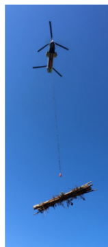
More than 5,000 logs were placed by helicopter in seven remote Yakima River tributaries...
