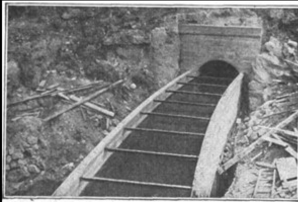
REINFORCED-CONCRETE FLUME BETWEEN TUNNELS
