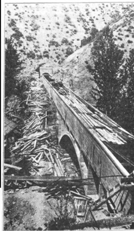
Fig. 1—Section of Flume Between Tunnels Showing Concrete Arch Built to Obviate Deep Excavation for Footings Across a Draw.
