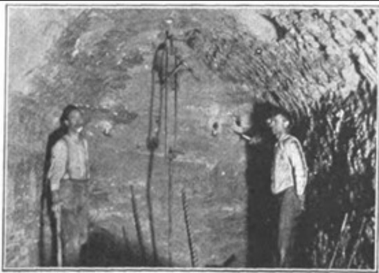
TUNNEL FACE SHOWING USE OF COAL AUGERS
