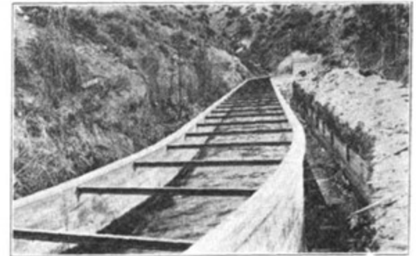
Fig. 2—Section of Flume, Cantilever Type, Between Two Tunnels, Making About a 10° Curve.
