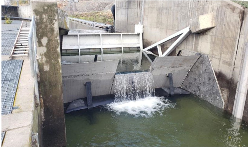
Sluice Gate Installation
