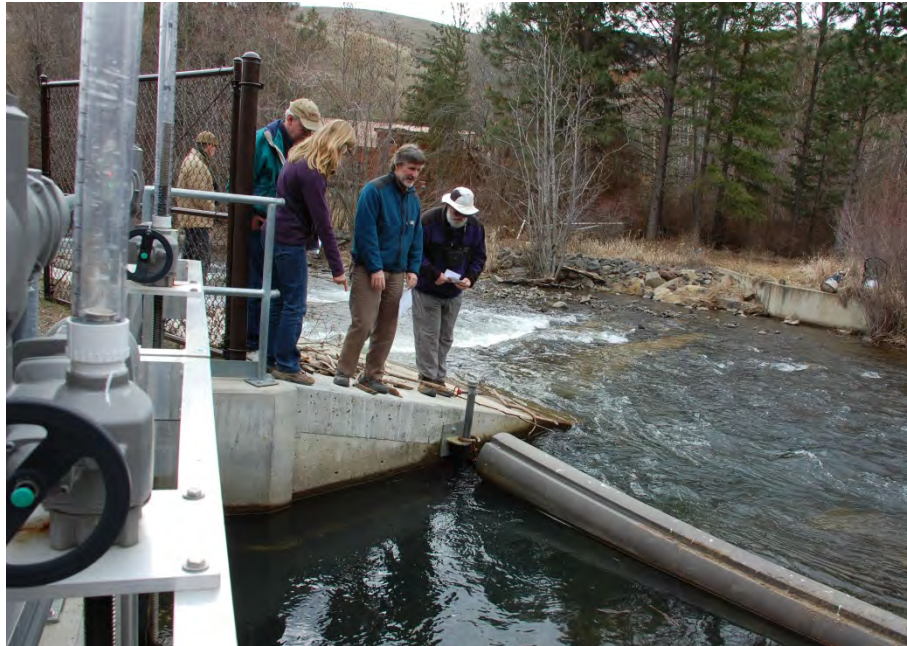
MWDA Diversion – Location of Transducer that is used to monitor streamflow
