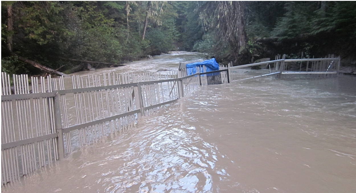
Figure 9. North Fork Tieton River fish trap after the high flow event on September 22, 2013 had partially collapsed the two weir panels on the right bank and weir pickets had been pulled to relieve pressure on the panels. The photo was taken the next day after the river had receded.
