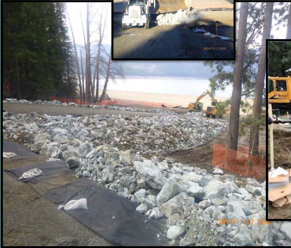
Installation of riprap along boat launch and vault toilet
