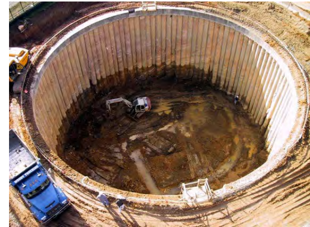
Secant Pile Example
