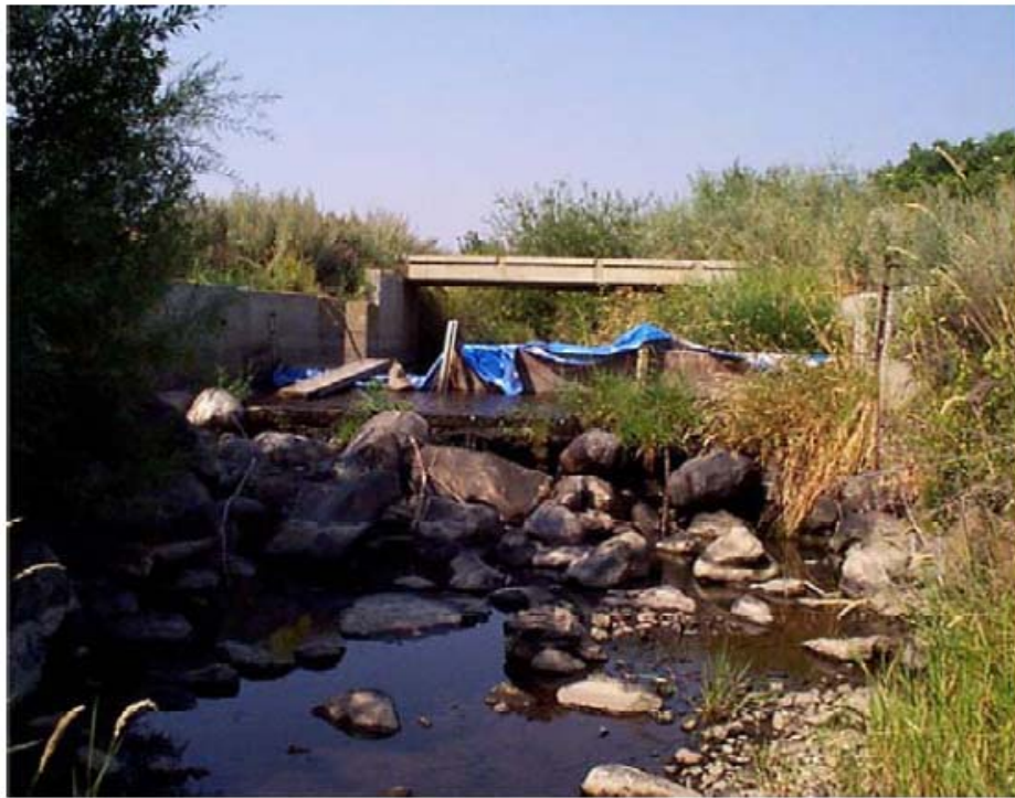
BEFORE: Irrigation dam blocks fish passage
