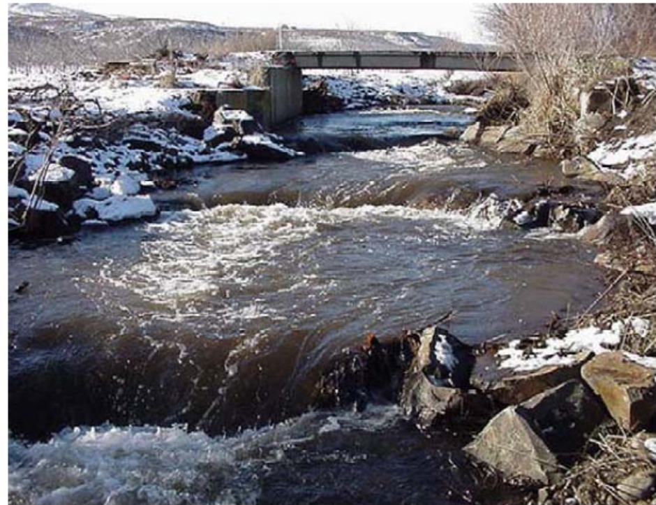
AFTER: Rock weirs allow full fish passage
