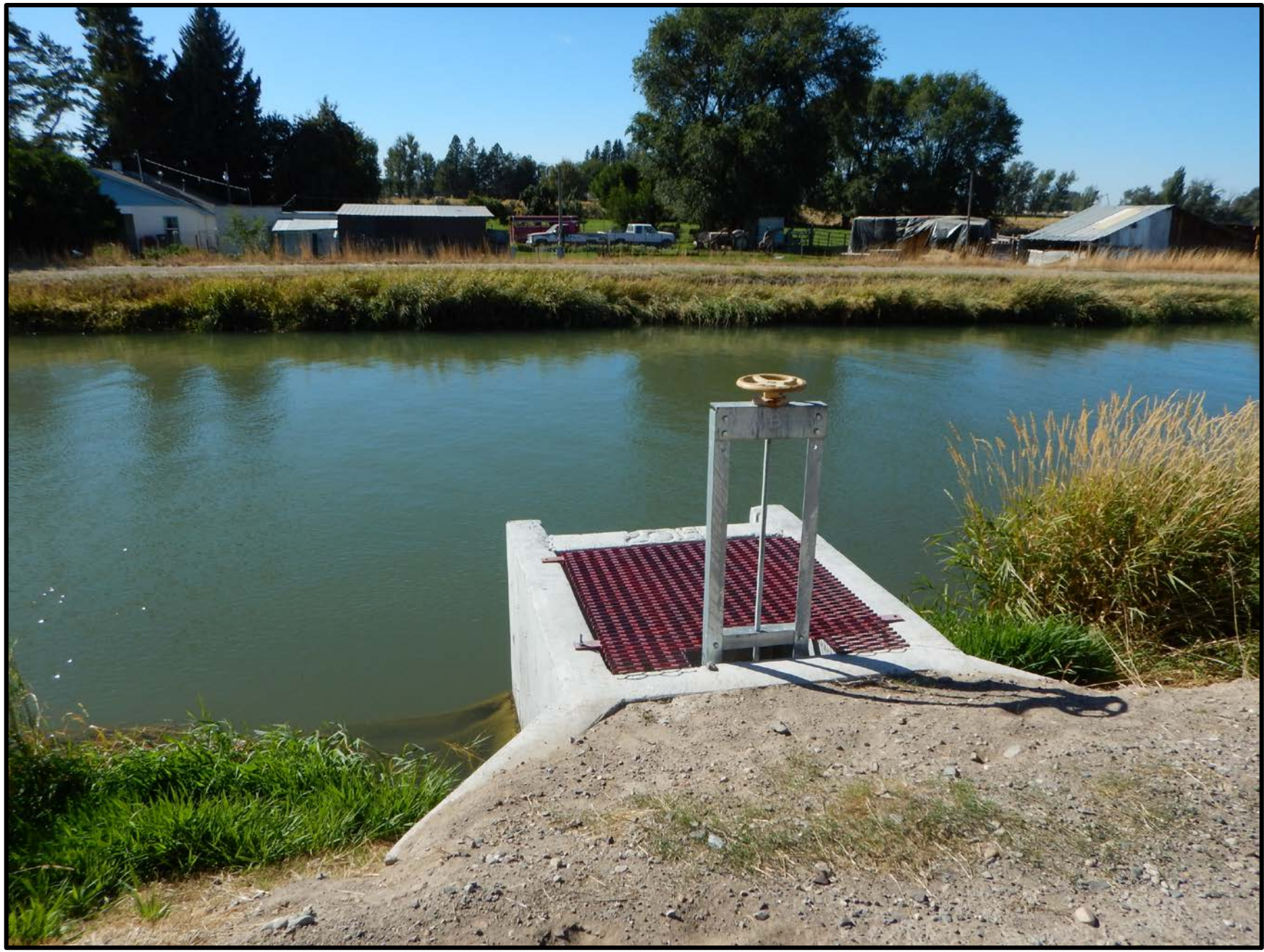
New turnout off of main canal into a lateral.
