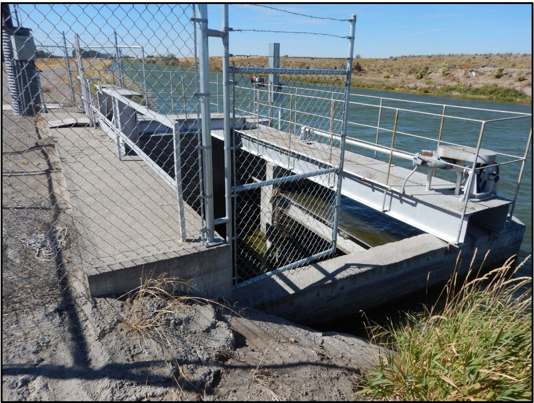
New control gates for the main spill off of the North Main Canal
