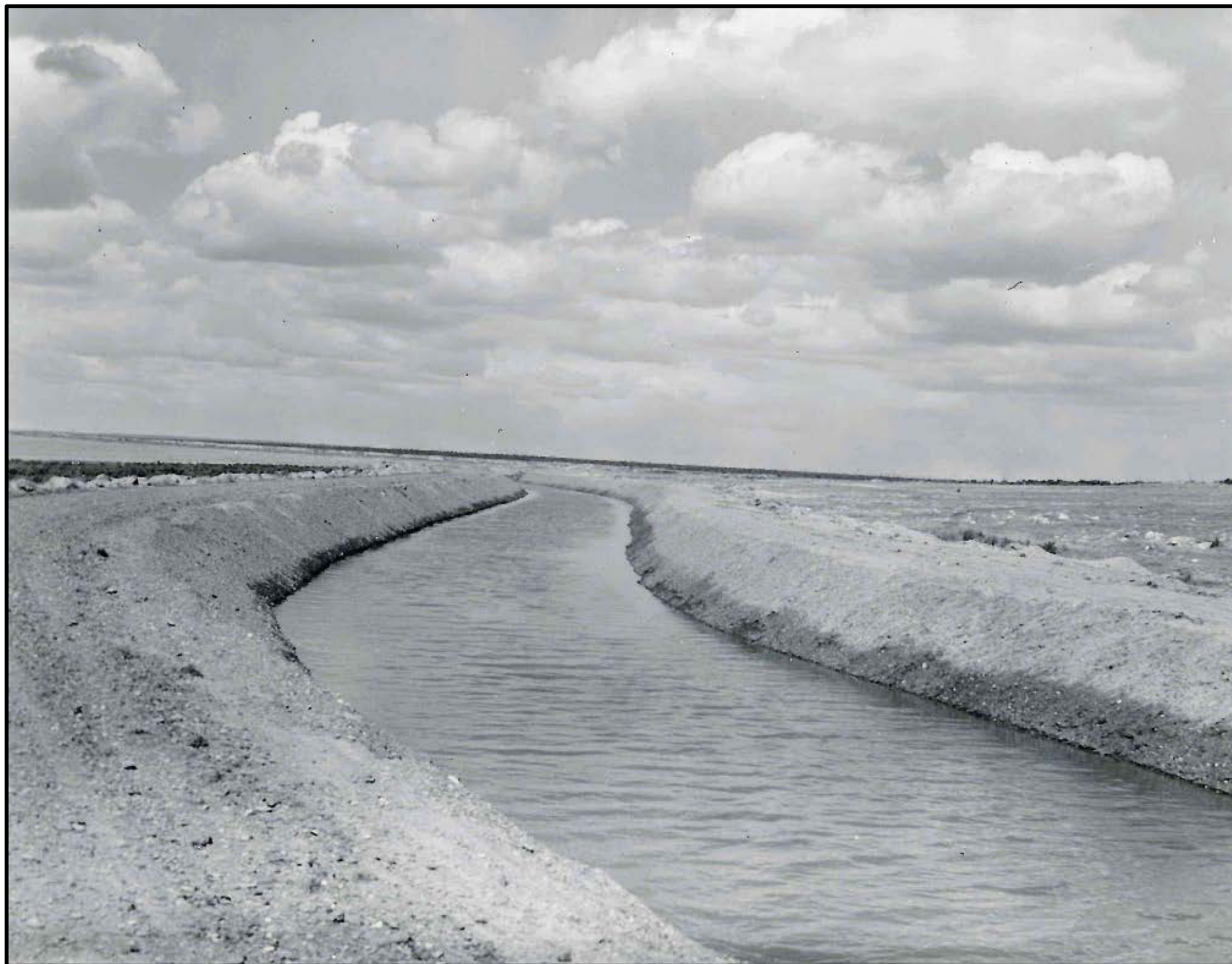
Photograph I-956. Unit "A" Main Canal, Showing Newly Constructed Dirt and Gravel Mixture Beach Belt. N.S.P.D., Minidoka Project – 1965. Courtesy A&B Irrigation District.
