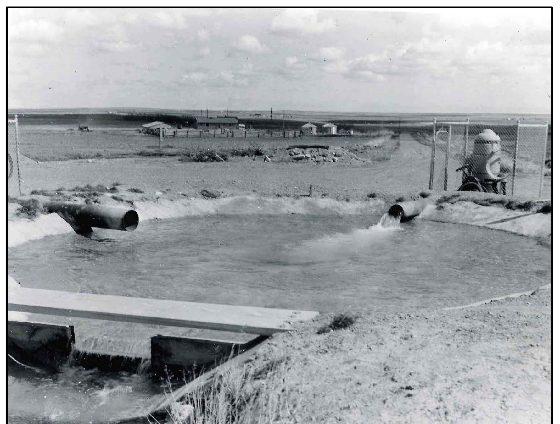
Photograph I-447. The 13AB 824 Stilling Pool Recently Lined with Concrete. This Pool Opened Up in the Bottom in 1955 and Took the Combined Discharge of Both Pumps, about 15 c.f.s. N.S.I.F.D. –Minidoka Project- May, 1960 – T. Gulley.
