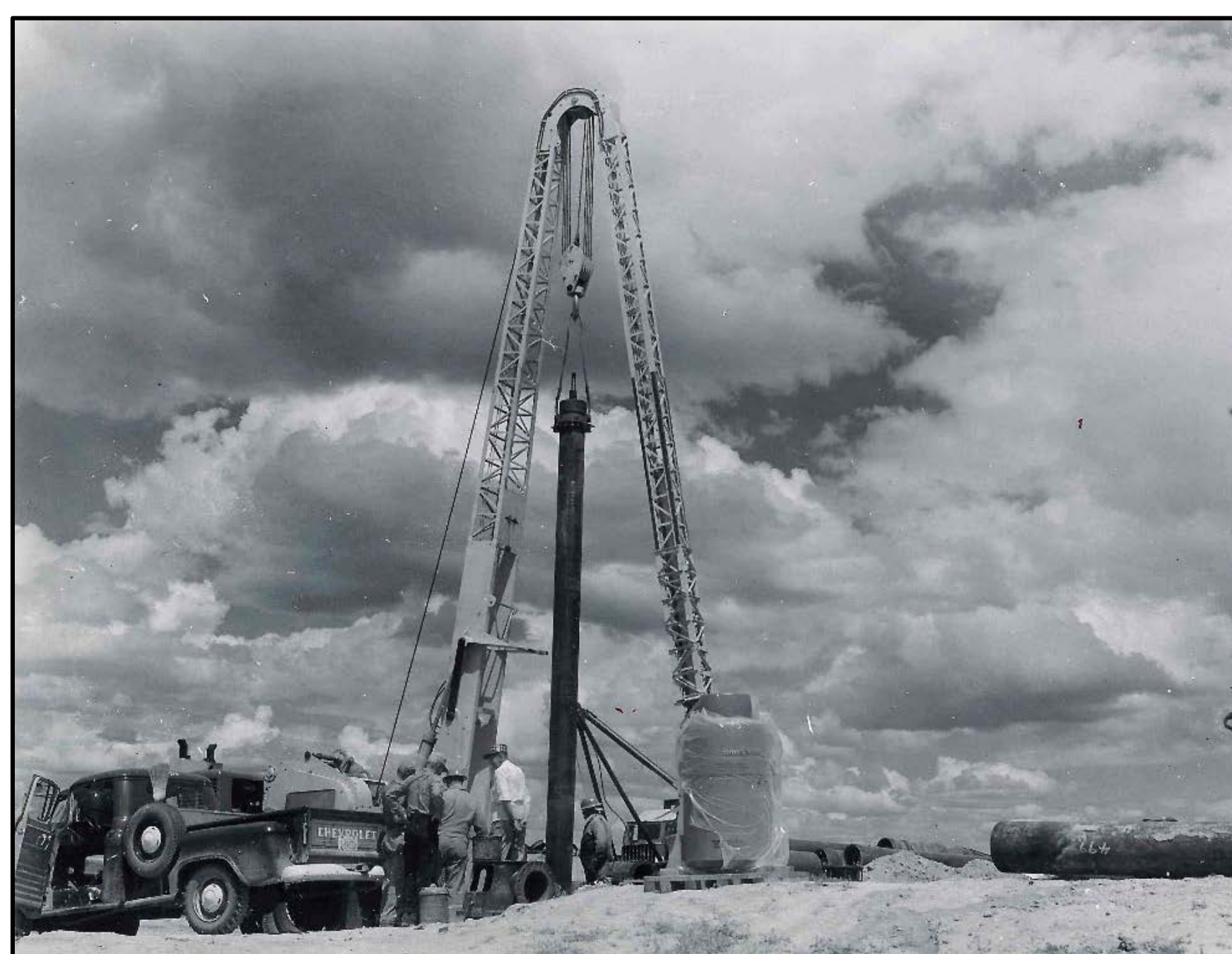
Photograph I-31. Installing 9A 922 in 33A 72 5 Well. June 1958, by T. Gulley.
