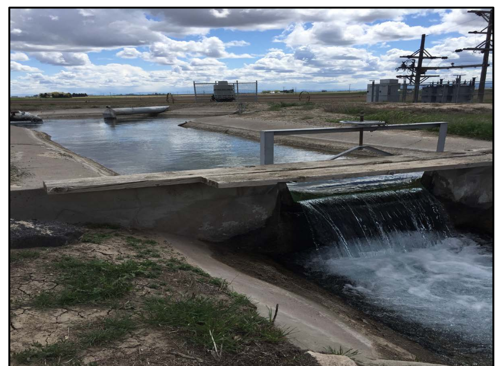
Concrete-lined Stilling Basin, with Lateral Extending to the West, View East.
