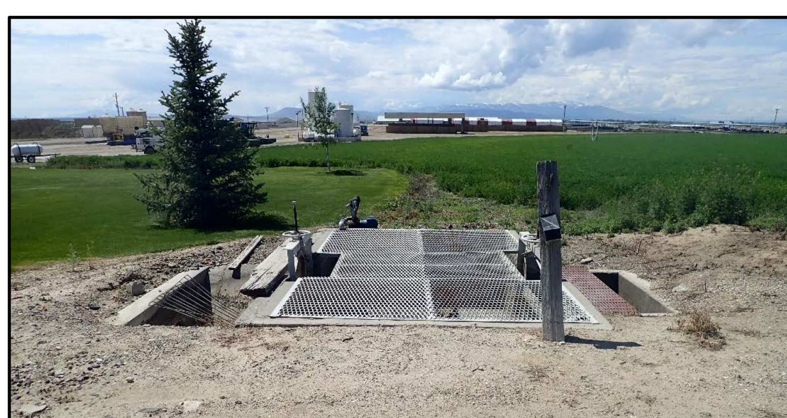
New Well Box Installed at 15AB825, View East.
