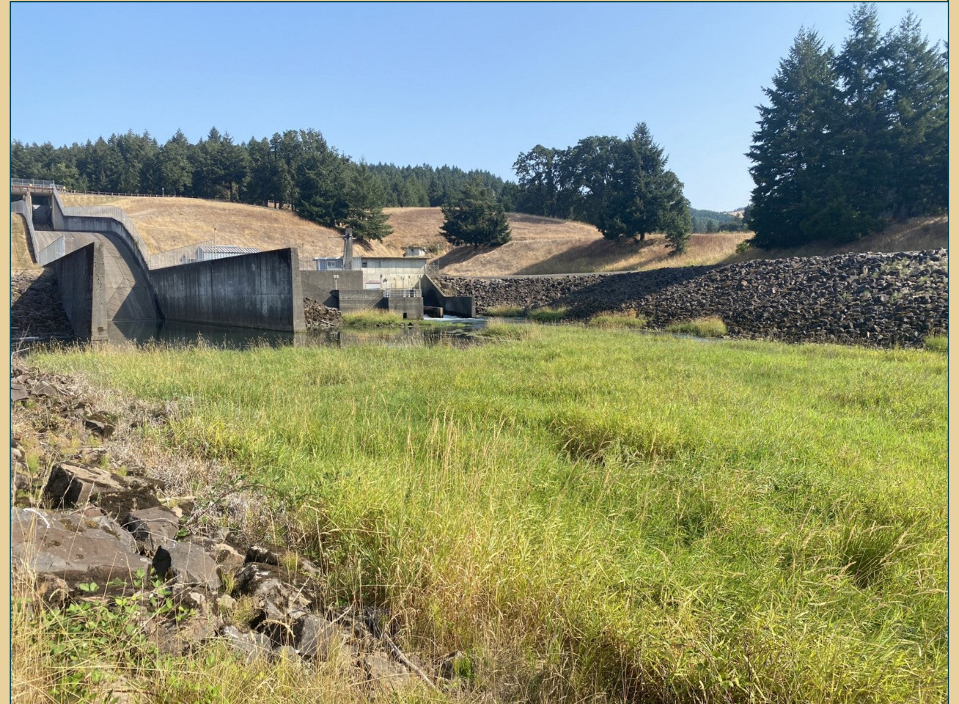
Image of Scoggins Dam spillway and outlet works. Photo Credit: Reclamation
