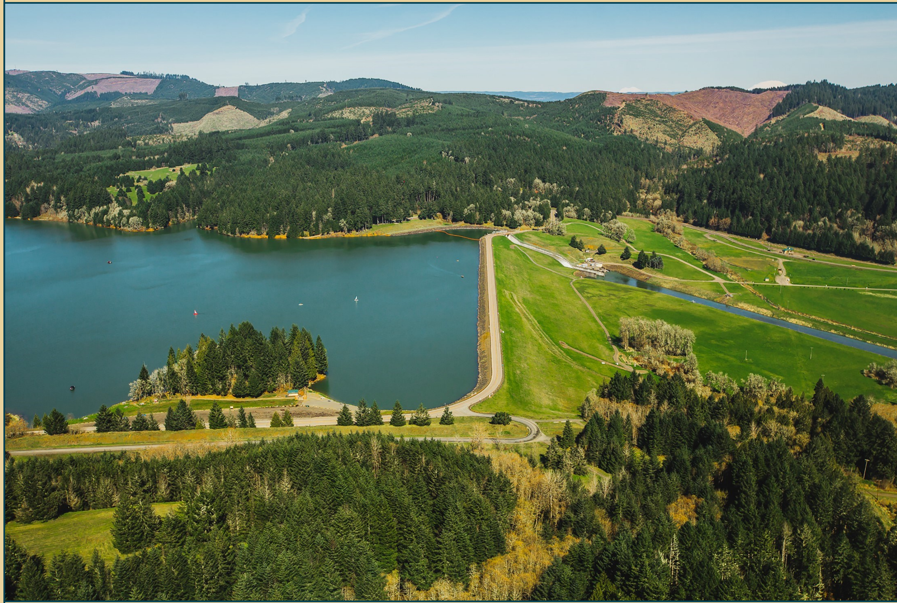
Aerial image of Scoggins Dam and Henry Hagg Lake. Photo Credit: Reclamation
