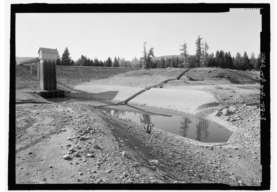
Photograph of upstream face of dam, gatehouse, tower, and inlet channel below buried conduit section, looking south at Kachess Dam taken by Thomas J. Wilson, 1992.
