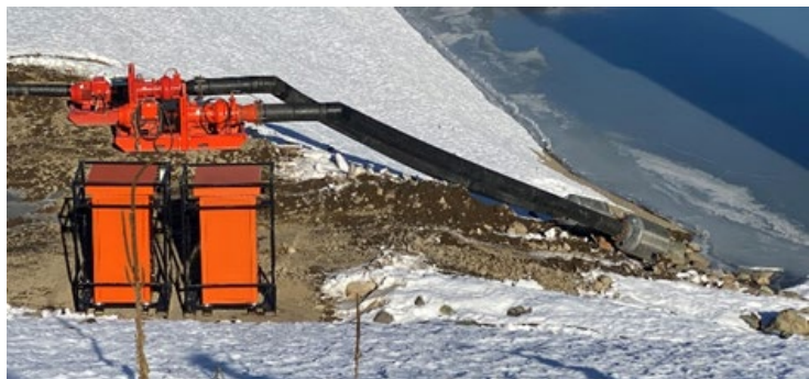
Figure 2-1. Land-based spillway pumps at Kachess Dam. Photo: Jason Sutter, Reclamation
