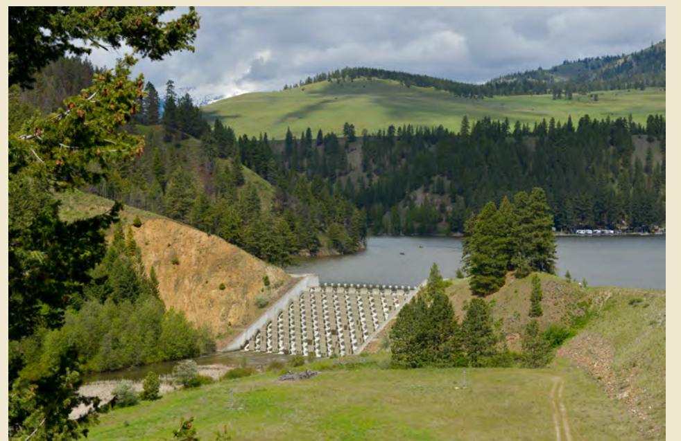
Conconully Dam, Washington
