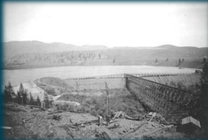
Material transported via flume to the damsite
