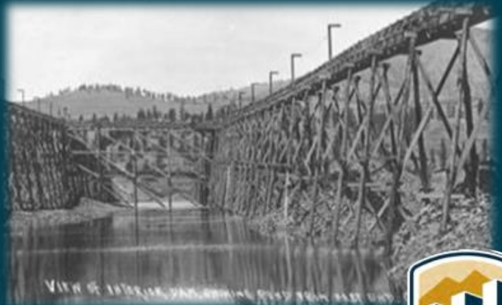
Hydraulic fill construction and puddled core
