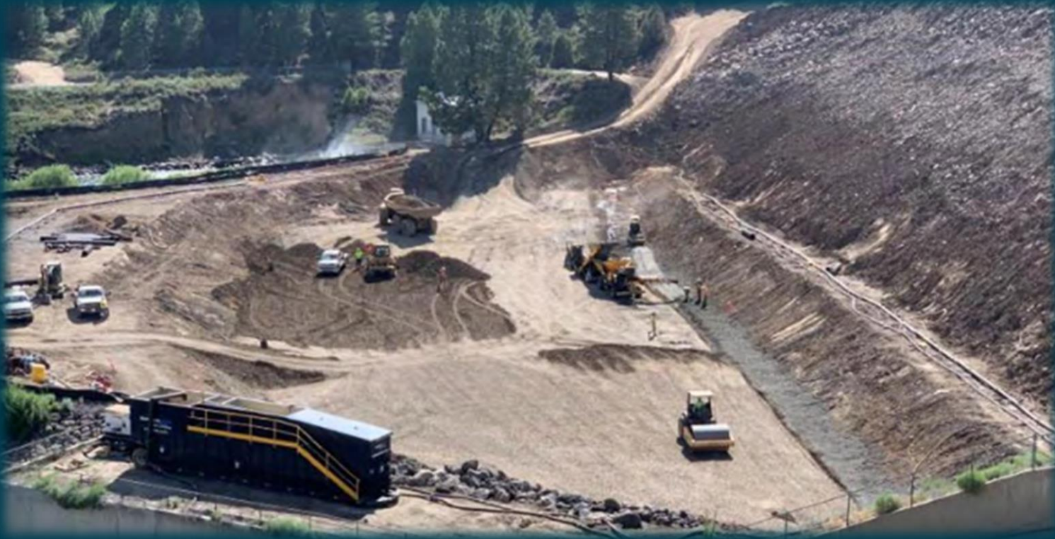
Excavate and replace implementation at Boca Dam.
